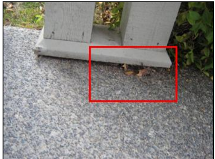
Loose due to concrete settlement
